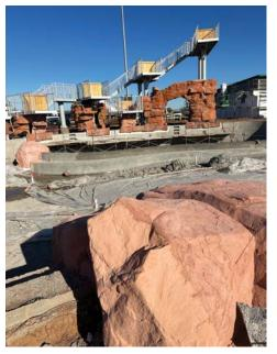
Left: Underwater and in-water boulders were strategically placed and finished with a hand-textured integral colour mortar to match the overall esthetic of the facility.
