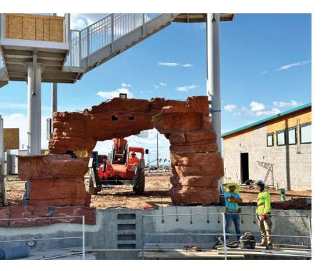
**Top:** A telehandler carefully maneuvered the rock segments into place around steel supports at the construction site.
