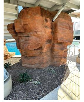
The completed faux rock formation highlights the detailed texturing and colouration that mimic natural geological features.
