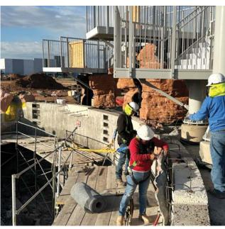
to the fabrication floor, where the foam cylinders were carefully spaced to match the layout. The steel framework was constructed around these foam cylinders, ensuring the dimensions aligned perfectly with the on-site requirements. This meticulous process proved successful, as the rock structures fit seamlessly during installation.
