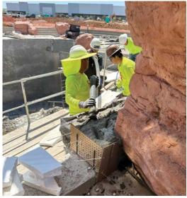
Arizona, for installation. The process began with concept drawings developed into a detailed vision over three to four weeks. A site visit was conducted to visualize the space and take precise measurements, which were used in Texas to lay out the structure on the fabrication facility floor and establish a sense of scale.
