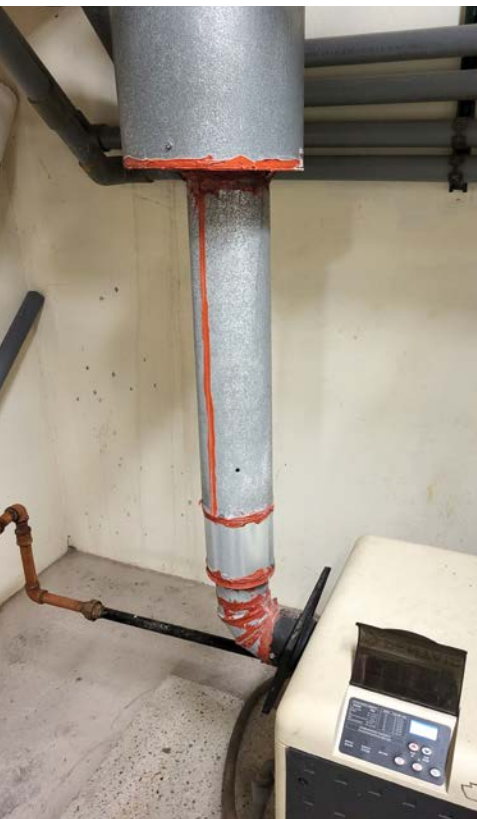
An example of improper vent material. This is a Category 3 positive pressure vent appliance with Category 1 venting for a negative draft appliance. The manufacturer calls for AL29-4C or equivalent venting.
