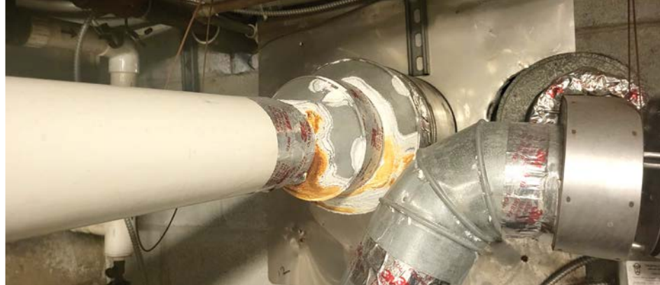
The manufacturer of this high-efficiency condensing pool heater specifies a polyvinyl chloride (PVC) vent system. Still, the installer ran PVC for about 1.52 m (5 ft) before transitioning into the existing vent system. The corrosion on the galvanized transition is indicative of condensate damage.
