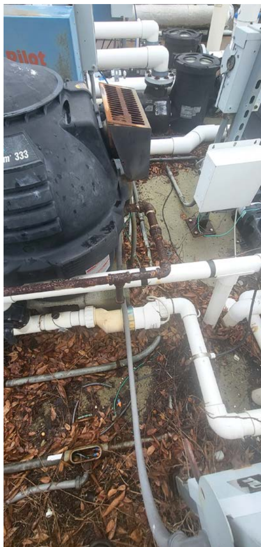
An example of undersized gas piping, and the heater is not installed per code and manufacturer specifications.
