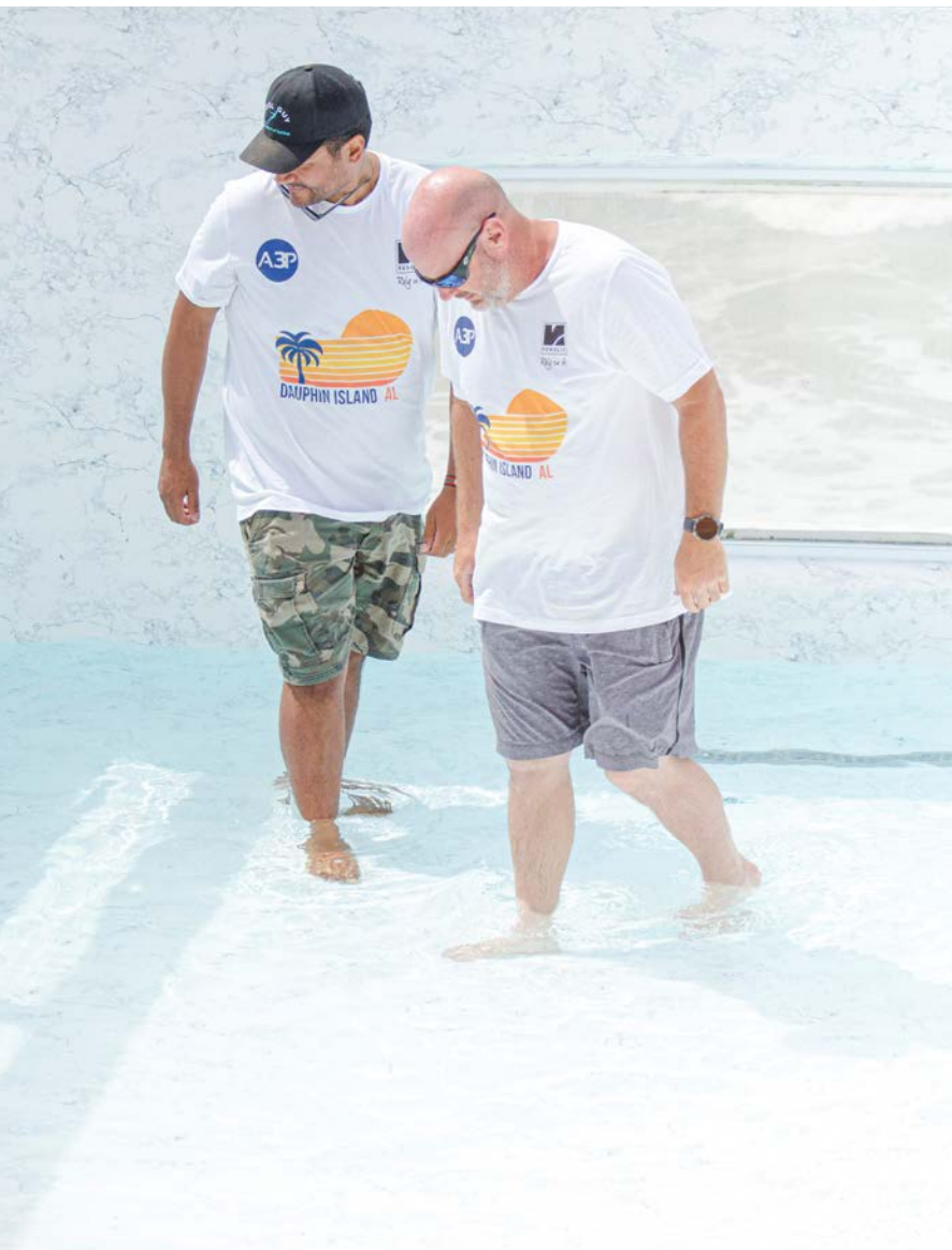
Two workers stand in a completed pool finished with a reinforced polyvinyl chloride (PVC) membrane.
