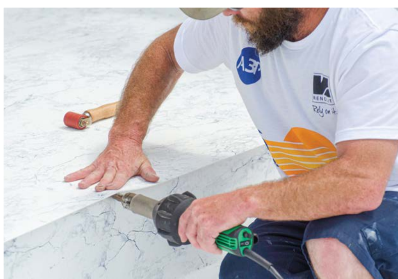
Top: Multiple crew members work together during the installation of a reinforced polyvinyl chloride (PVC) membrane.
