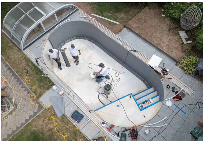
Reinforced PVC membranes are installed as welded interior systems that create a continuous, watertight surface across the pool structure.
