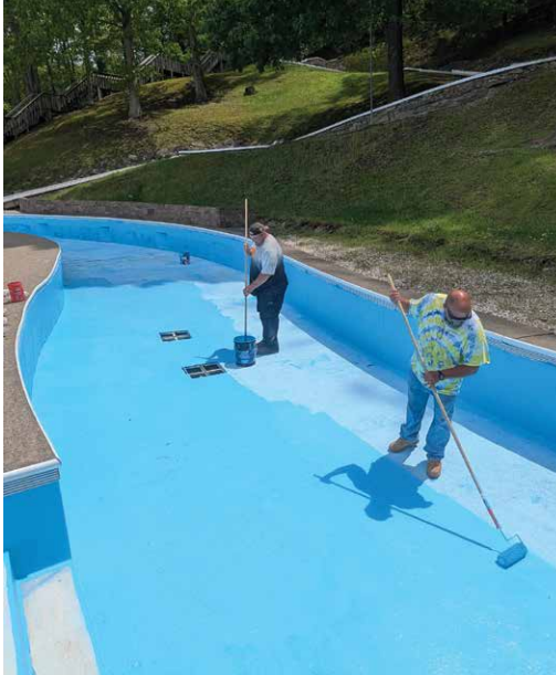
Concrete coatings can be applied quickly and easily.
