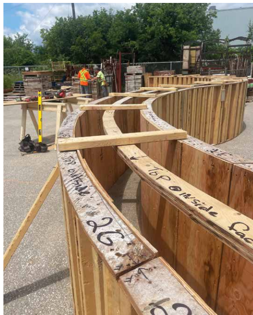
By prefabricating the curved formwork sections off-site, it reduced labour requirements and helped to maintain dimensional accuracy.
