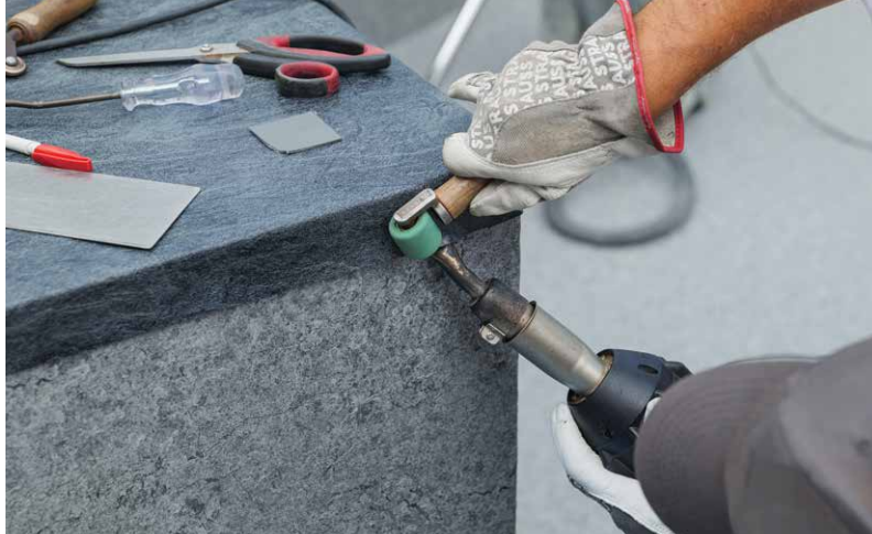
Reinforced PVC membranes are installed as welded interior systems that create a continuous, watertight surface across the pool structure.
